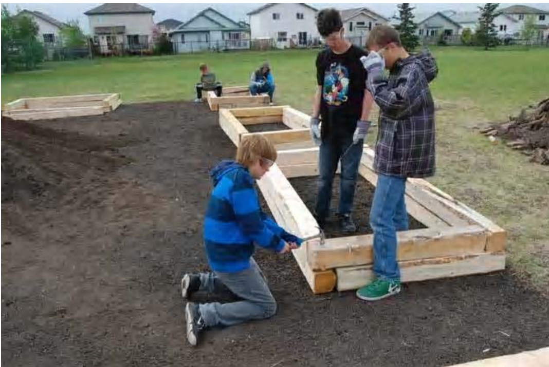
All the older students took turns building!
